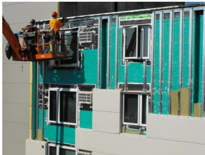
FIGURE 5. Shows the liquid WRB over original brick with fire resistant insulation, new windows and super insulated metal panel installation
