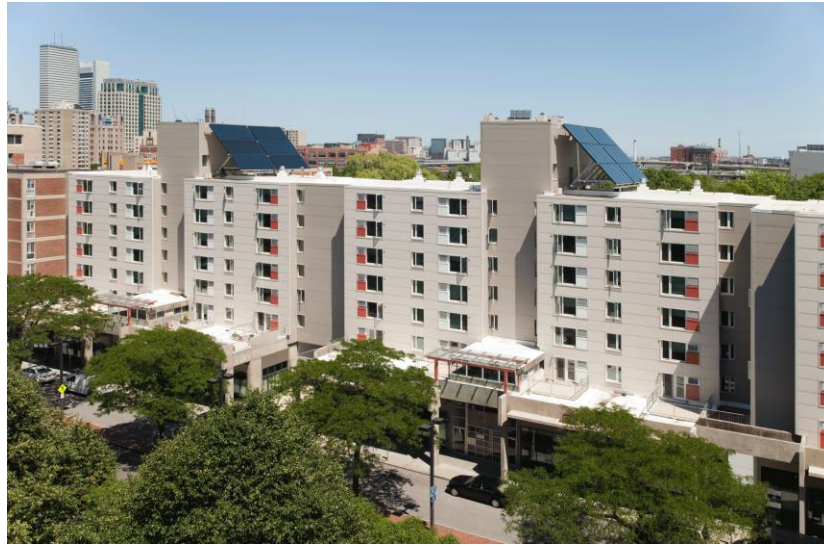
FIGURE 7. Castle Square Mid Rise Units with Super Insulated Cladding, new R-5 Windows , Highly Reflective TPO roof with additional insulation and Solar Collector for hot water
